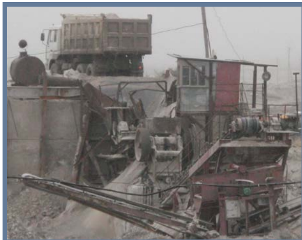
Safety issues at the ZhambylGips rock crusher
