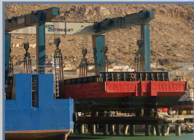
EBRD style ESDD and ESA of MOBY BOAT YARD Construction
