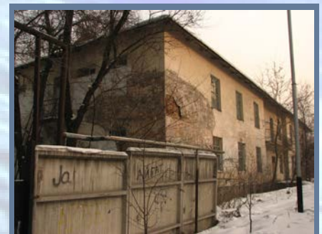
Old residences at Satpaeva Mixed use complex, Almaty required resettlement
