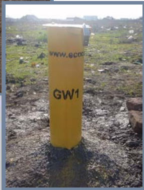
Finished wellhead
