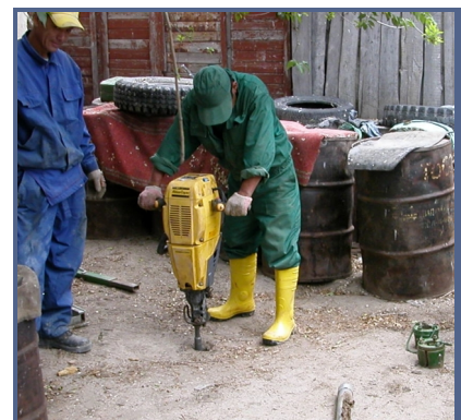
Unlined fuel drum storage
